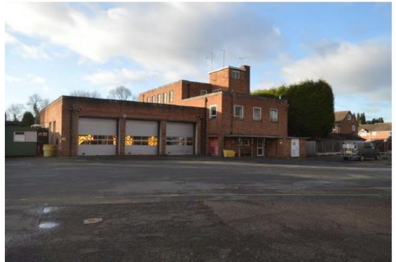
View WNW of E Elevation of Redditch Fire Station
