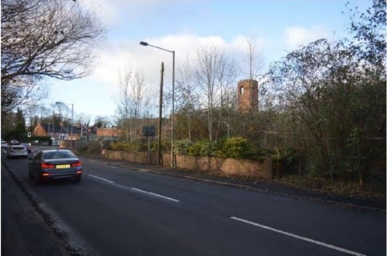
View NW from Middlehouse Lane (Training Tower visible)
