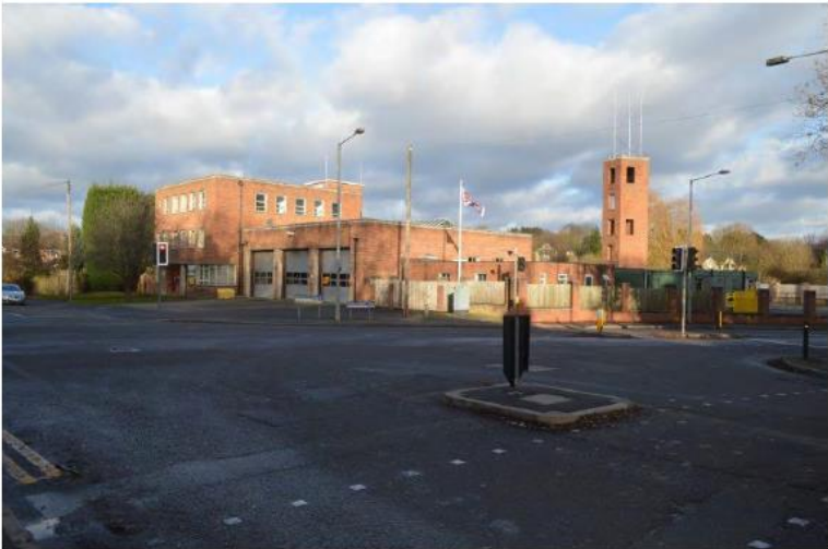
View NNE of Redditch Fire Station from Junction of Birmingham Road and Middlehouse Lane
