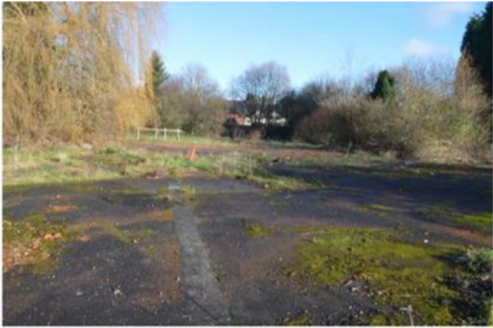
View NE over hardstanding in E part of Site
